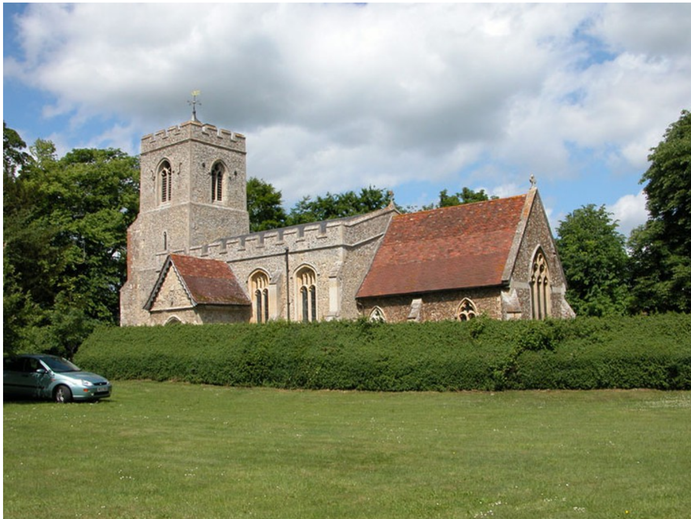
Ext. general view from SE
