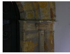
Two orders, round-headed. The two arch orders are plain and square in section with a keeled roll label with short returns at the ends. First order (jamb). Chamfered with plain stops and slender hollow-chamfered imposts, quite plain and partly replaced. Second order (jamb). Cylindrical en-delit nook-shafts on low roll bases with thin roll neckings. The bases stand on raked plinths. Both capitals are stiff-leaf with roll neckings and the imposts are of the same profile as the first order.
