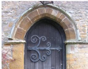
Single order, pointed. The arch and jambs are chamfered, and the arch springs from impost blocks that are hollow chamfered with an overhanging face carved on its surface with a low roll between quirks.
